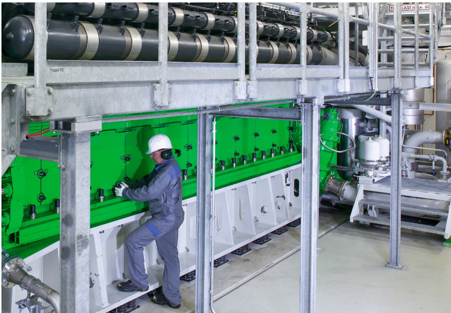
GE's 10 MW class J920 FleXtra engine is part of the Stadtwerke Rosenheim municipal cogeneration plant in Germany
