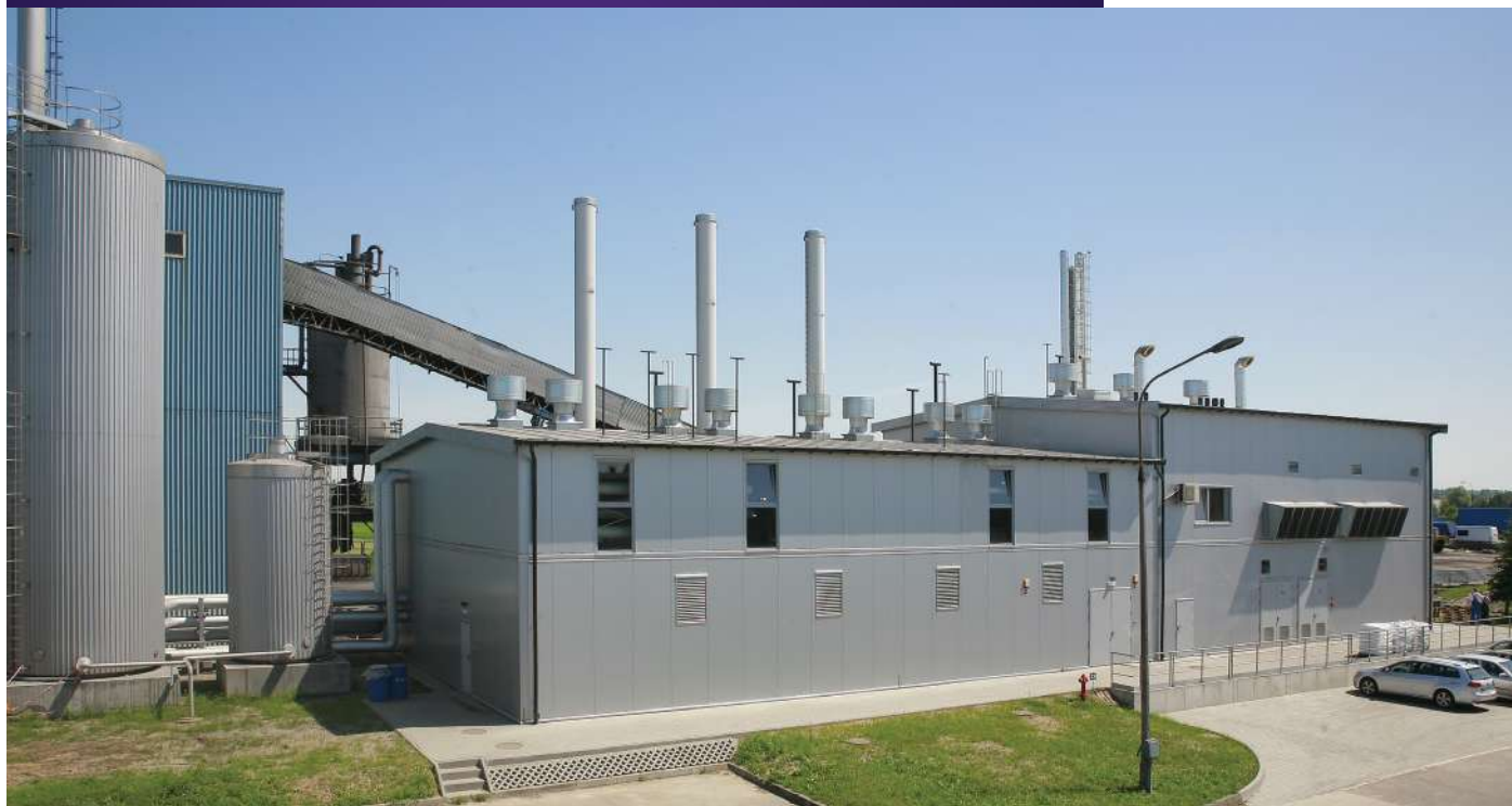
Condensation plant - Sokołowie Podlaskim - Poland.
